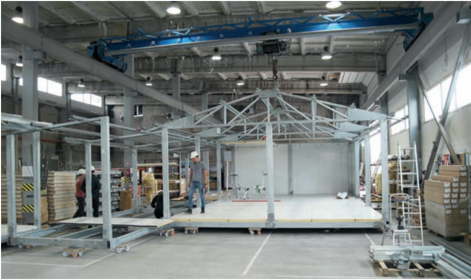
Trial erection of the school at a Combiworks network factory.
