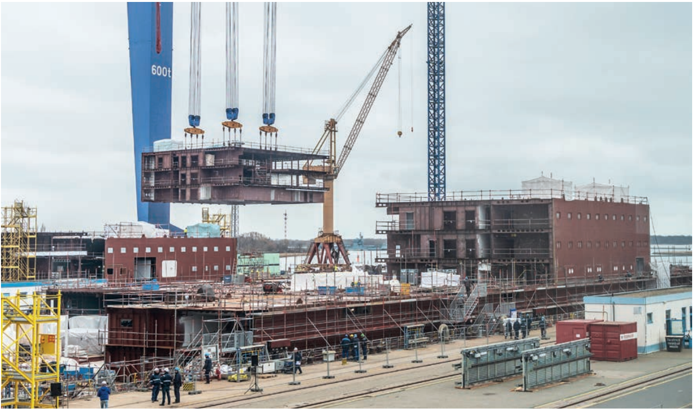
Building progress: On 1 March 2019, section 50 was lifted into the dock at the Rostock-Warnemünde yard.
