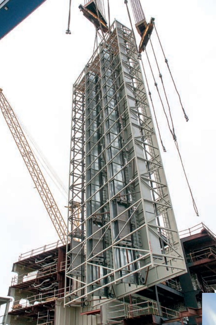
▲ Installation of a drop-in elevator trunk module
