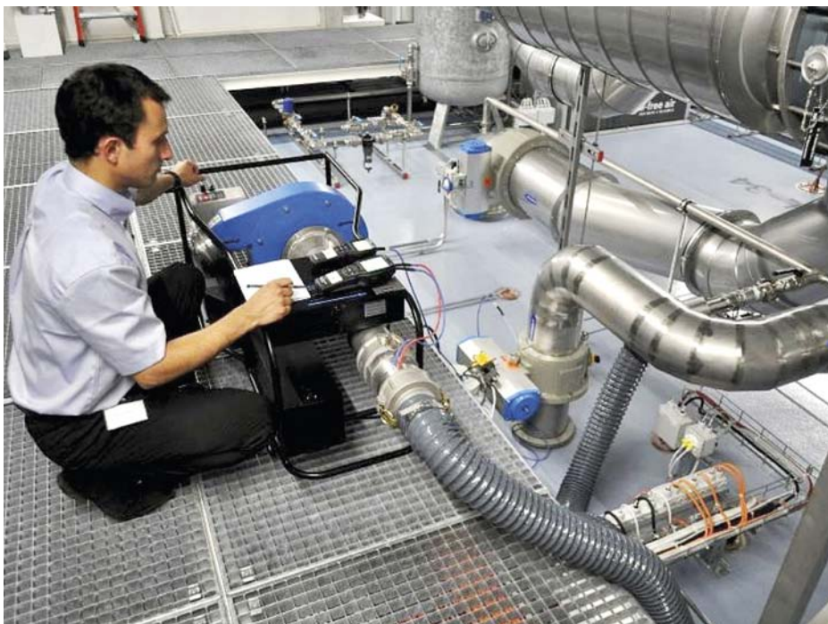
◀ Room impermeability tests
