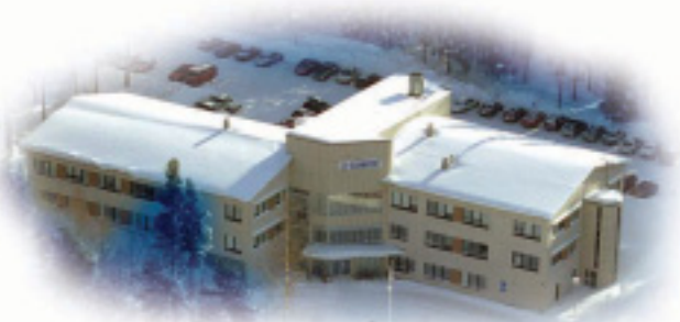
Real estate energy audits reduce costs through energy savings
