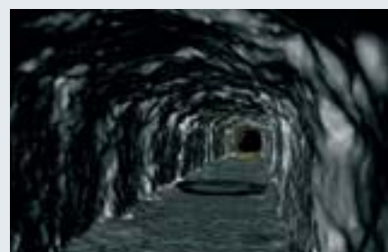
Field and tunnel surveying
